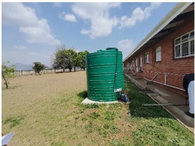
Photo 04 – Showing ‘JoJo’ tank storage with associated water pump and pipe connections.
