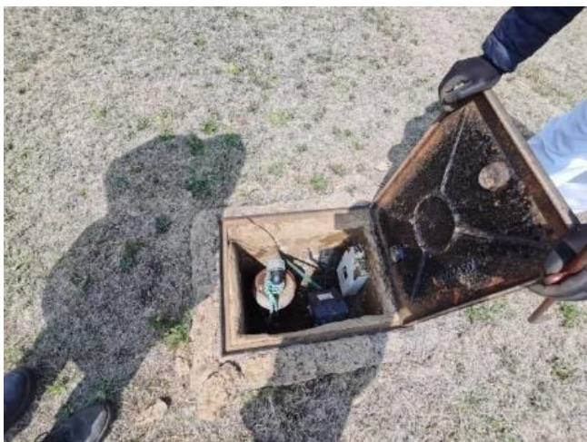
Photo 03 – Showing typical borehole and associated components.
