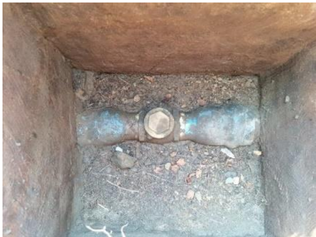
Photo 02 – Showing non-return valve.
